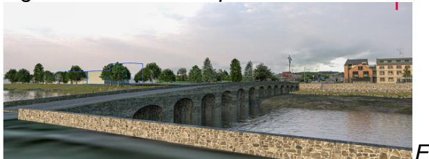
Figure: View from footpath to the north of the Long Bridge
